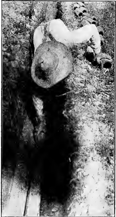
FIG. 83. Laying double-sole drain-tile by hand.
